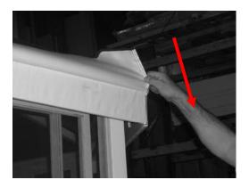
Once the vinyl roof is properly centred and the sewing seams are well aligned with the rafters, pull down each corner of the vinyl roof over the cornices as seen on the picture below.
