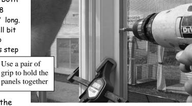
Now you are ready to install the cornice on top with 5/16" self taping screws. The holes have been predrilled at the factory for your convenience. The cornice must be flush and equidistant to each corner as seen in the picture below. Each cornices are as long as two panels edge to edge.
