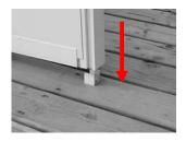
• Install the second panel, fix both panel together with three #8 square head metal screws of 3" long. Pre-drill one of them with a drill bit 5/32" inside the window lock to conceal the screws. Repeat this step 3 times
