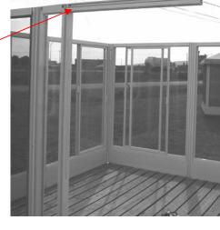
• To fix the second panel, measure 35 inches from the previous panel (this is the required opening for the door), and install a U bracket on your platform as shown. When the bracket is well positioned, insert the panel and fix it with 5/16" self taping screws.
